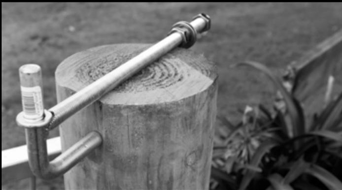
When mounting gates to timber strainers it's best to use Through Post Gudgeons, which go all the way through the strainer for extra strength and adjustability. Greyson or Franklin Lock Thru Post Gudgeons (with a hook-like 'locking tail' under the pin) are a good choice as they won't twist in the strainer. Each gudgeon needs to be long enough to easily pass through the centre of the strainer, comfortably allowing enough excess to attach and adjust the outer nut.
