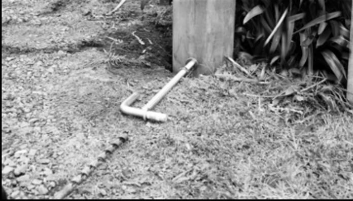
The gap between the centre of the top gudgeon hole and the centre of the bottom gudgeon hole should match exactly the distance between the hinges on the gate. Drill this hole on the same angle as the top gudgeon (positioning the gudgeon on the ground as a guide may help). Again, check that the drill bit is horizontally level before you start drilling. Insert the gudgeon, mark and drill the hole for the locking tail. Insert the locking tail and hand-tighten the gudgeon's outer nut.
